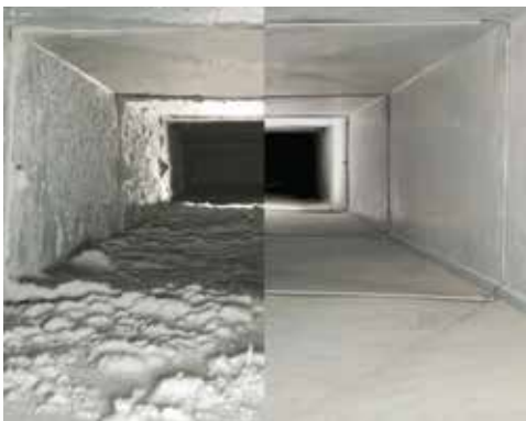
Ducting before and after cleaning.
